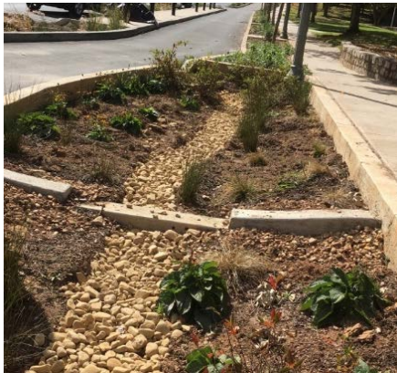
Green infrastructure – like this installation on McDonough Street – is an important part of Decatur’s SWMP.
