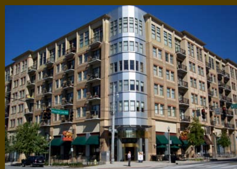
DENSITY BONUSES Developers provide a number of affordable units in exchange for greater allowable density.
